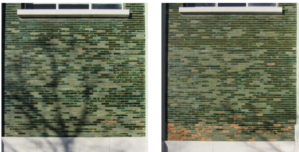
Figure 4: Casa da Moeda , Lisbon. Left: preserved as originally; right: decayed at bottom.
